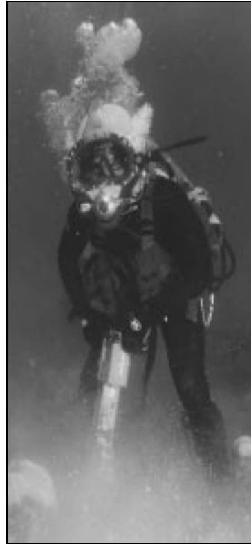
Figure 6-4. Underwater Construction Diving.
